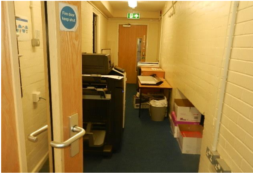
Figure 11: Internal access corridor to administrative area.
