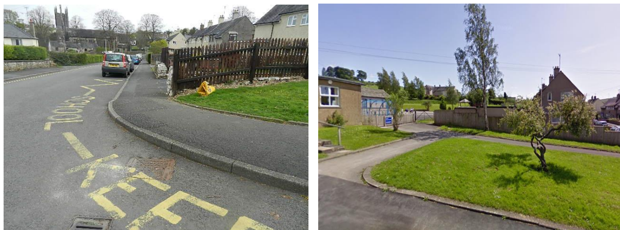
Figure 4: View of pedestrian approach routes to the school.
